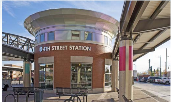
Reno's 4th Street Bus Station, Reno Nevada
